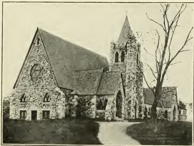
No. 27 ALL SAINTS' EPISCOPAL CHURCH, CHELMSFORD CENTRE
